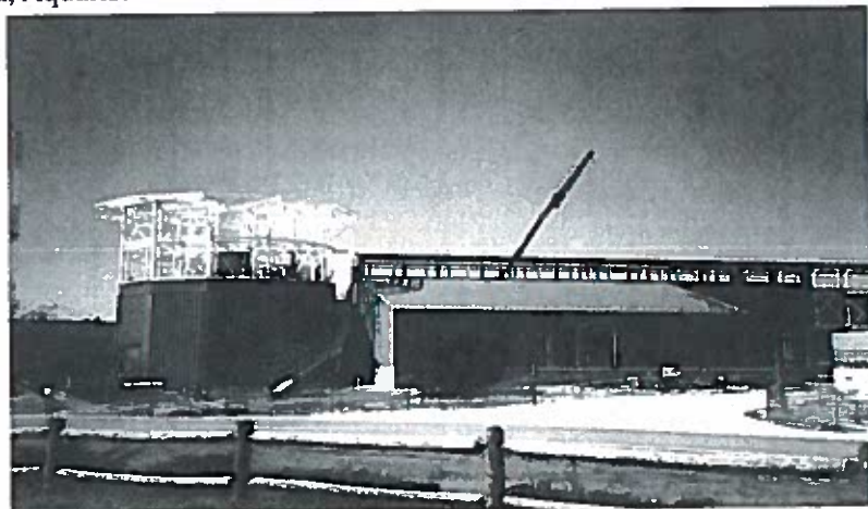
The Estuarium during construction.
